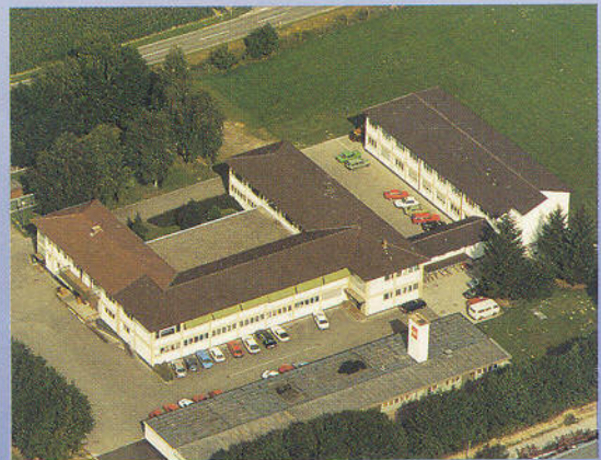
BARCO-EMT company site in Kippenheim
